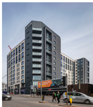
PERSHORE ROAD, BIRMINGHAM for: Hallmark-By Developments Ltd 330 Units / £36m / Completed 2018
